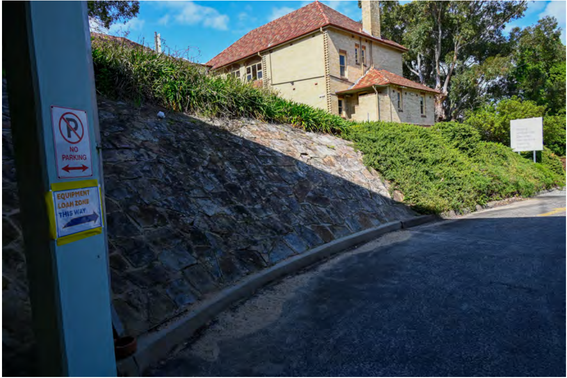
Internal access road from River Road. Heading south. Area of 'Service and deliveries'.
