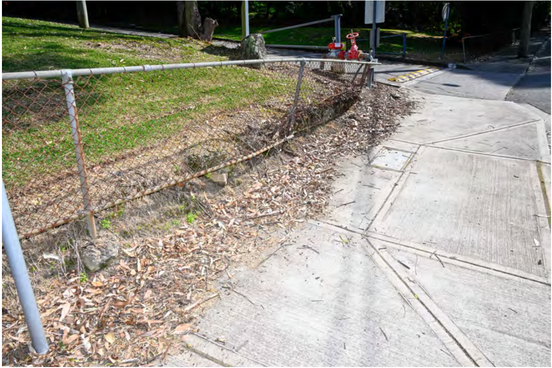
Hospital access from St Vincents Road. Western side of the road. Area of the pedestrian crossing. Damaged fencing.
