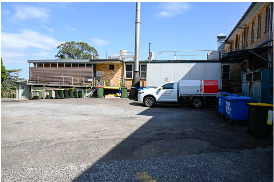
Internal access road. Heading south. Area of 'Service and deliveries'.
