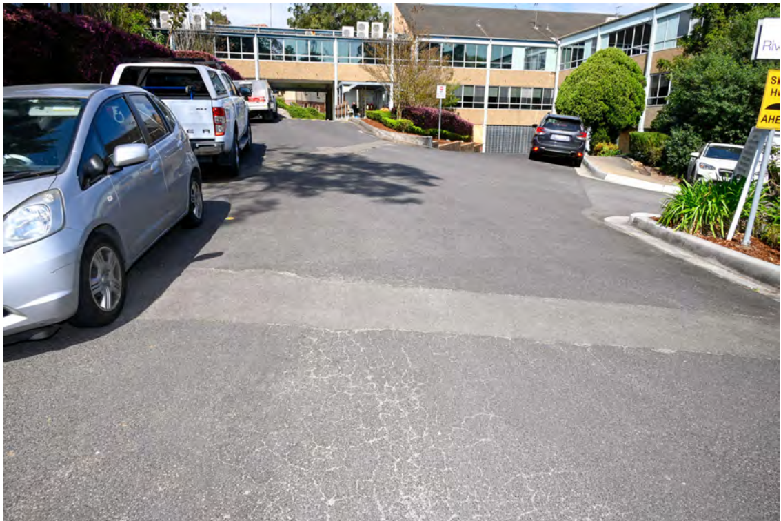
River Road. Area of the proposed substation works. Internal access road. Cracked and crazed state of the road paving.
