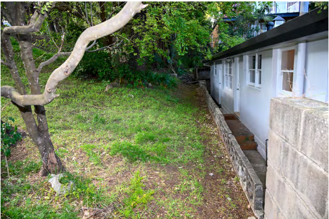
Southern property boundary. Heading east towards St Vincents Road. Common boundary with 24 Gore Street.
