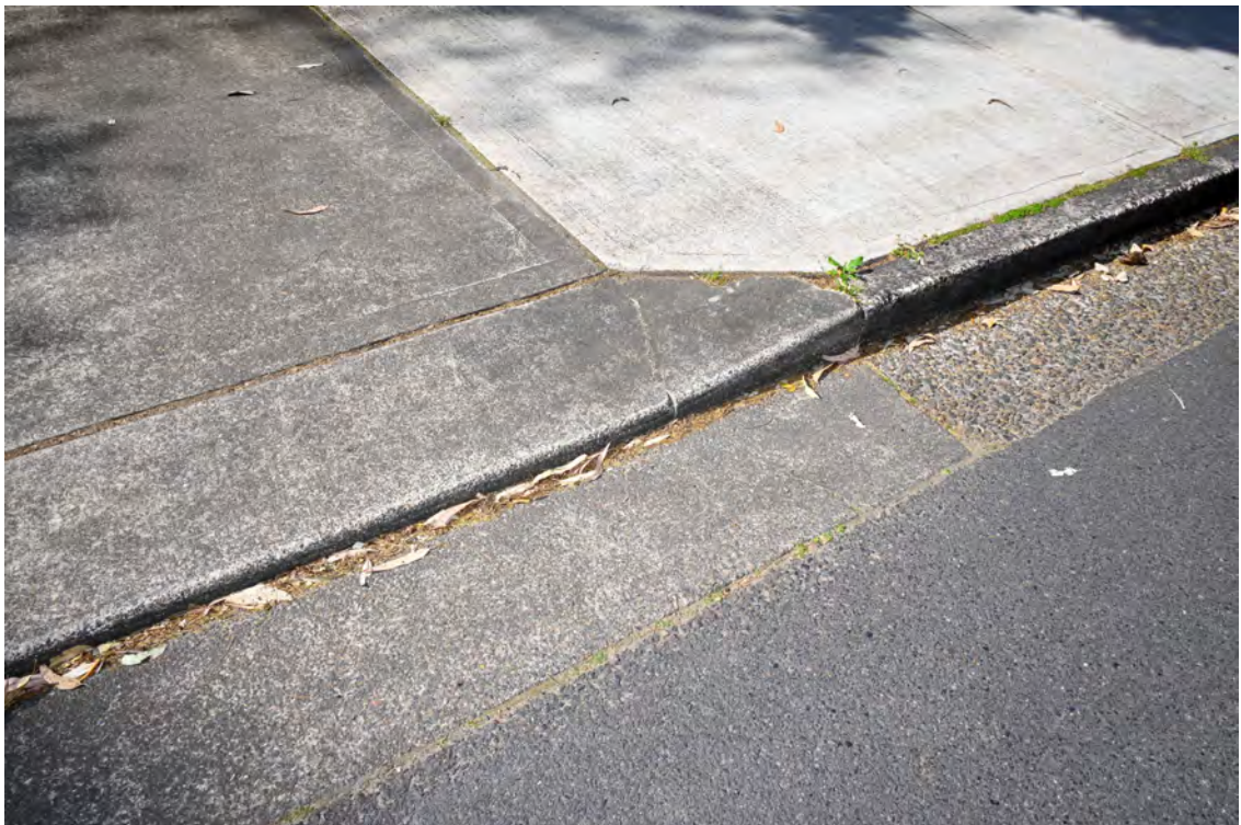
Hospital access from St Vincents Road. Area of power pole no. GL72349. Eastern side of the road. Heading south. Crossover to 18 St Vincents Road. Cracked shoulder of the layback.
