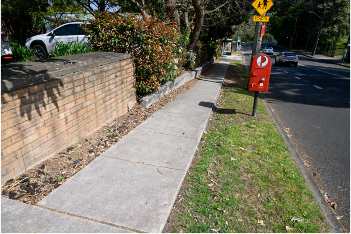
Hospital access from River Road. Area of the proposed substation works. Western side of the intersection. Heading west. Area of the 'Sprinkler Booster'.
