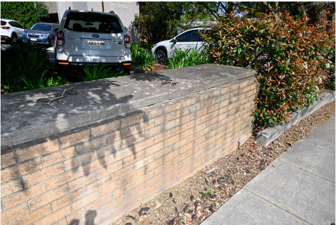
Hospital access from River Road. Area of the proposed substation works. Western side of the intersection. Heading west. Area of the 'Sprinkler Booster'.
