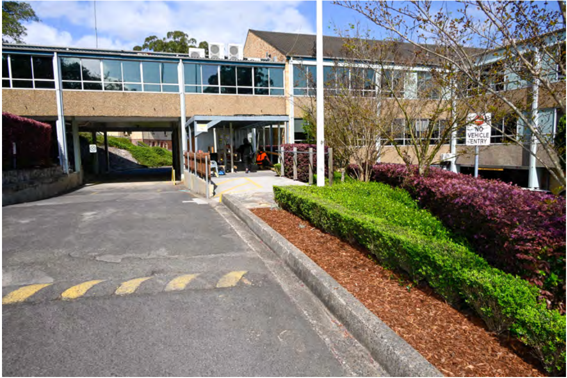
Internal access road from River Road. Heading south approaching the overhead walkway.
