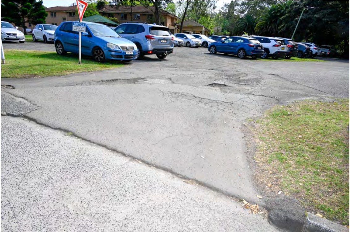
Hospital access road from St Vincents Road. Area of Pallister House. Adjacent parking area. Damaged asphalt paving.
