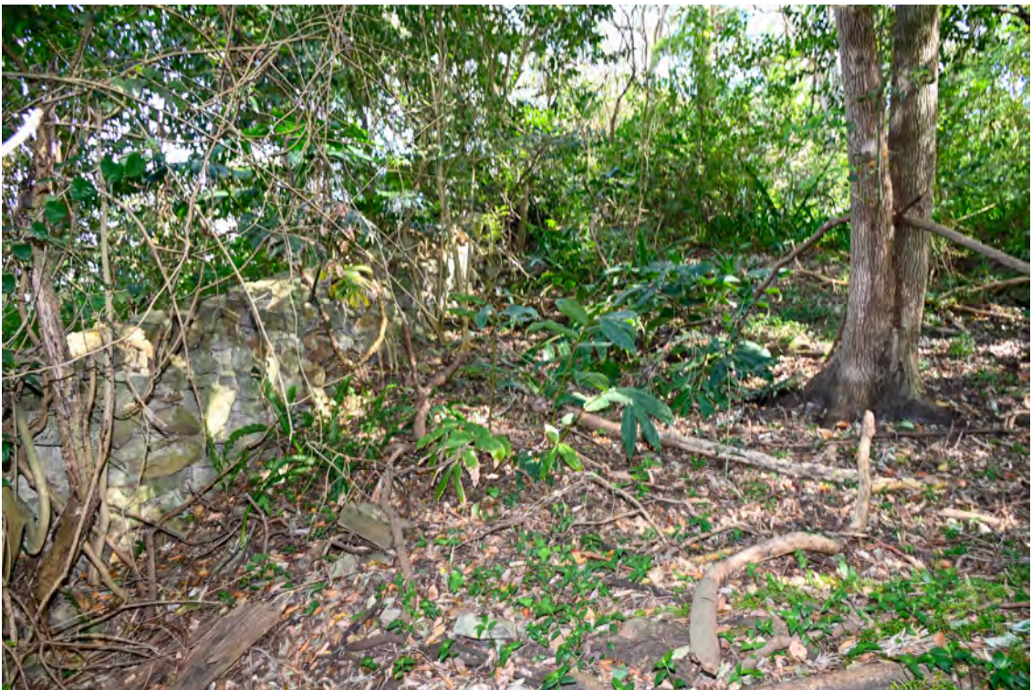
Southern property boundary. Area of the common boundary with 39 Gore Street. Heading west.
