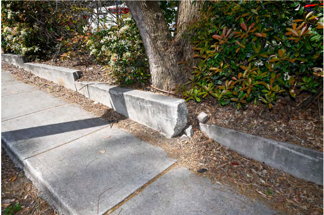
Hospital access from River Road. Area of the proposed substation works. Western side of the intersection. Heading east. Area of the 'Sprinkler Booster' and power pole no. GL72380. Damaged retaining wall.
