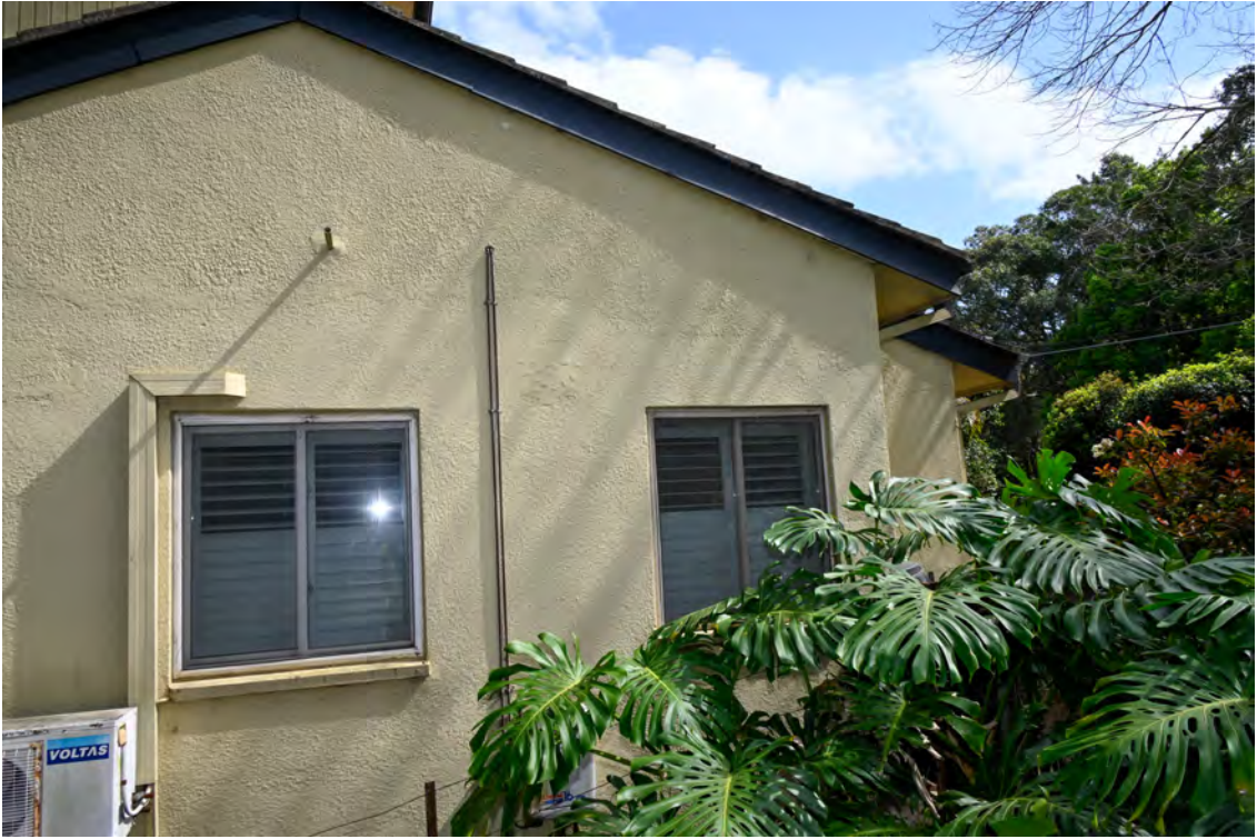
Western hospital boundary. Heading south. Area adjacent to the common boundary with 117 River Road.
