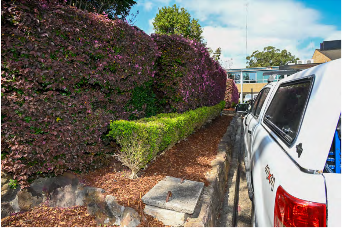
River Road. Area of the proposed substation works. Area on the eastern side of the internal access road. Record of the landscaping.
