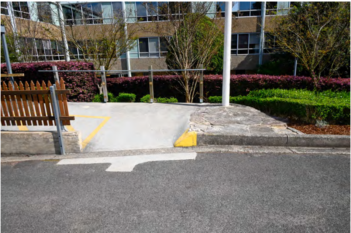
Internal access road from River Road. Heading south approaching the overhead walkway. Western side of the road.
