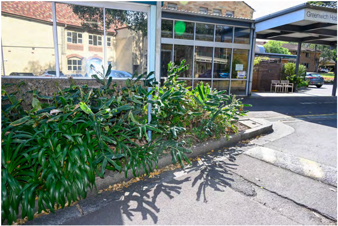
Internal road between Pallister House and 'Health & Care'. Heading north-east / uphill. Area of proposed road works.
