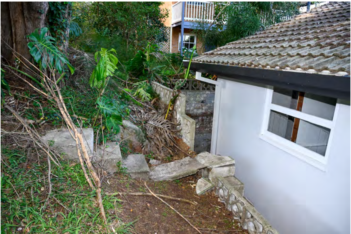
Southern property boundary. Heading east towards St Vincents Road. Common boundary with 24 Gore Street.
