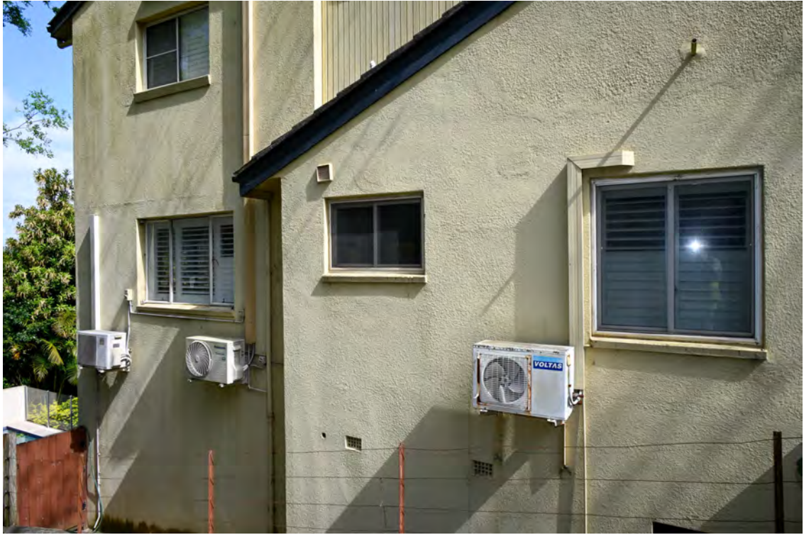
Western hospital boundary. Heading south. Area adjacent to the common boundary with 117 River Road.
