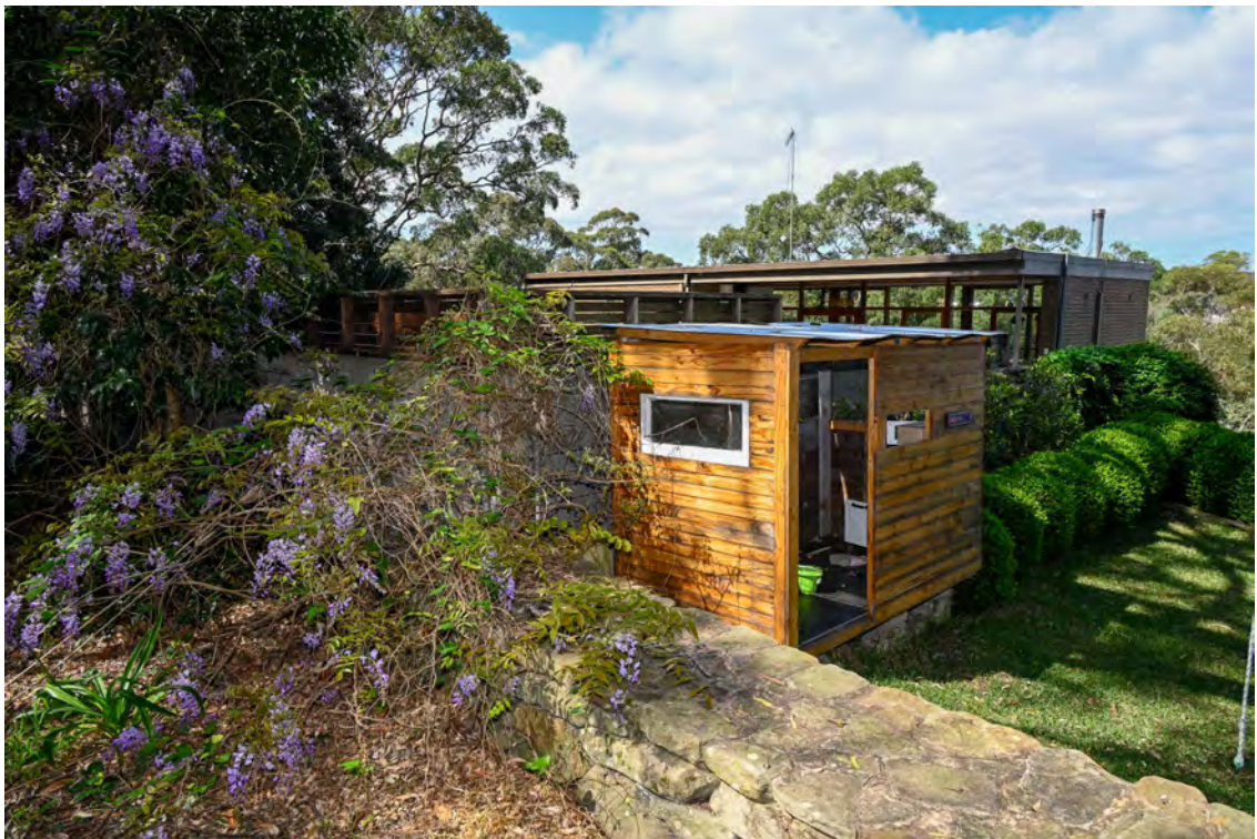
Southern property boundary. Heading east towards St Vincents Road. Common boundary with 51-47 Gore Street.
