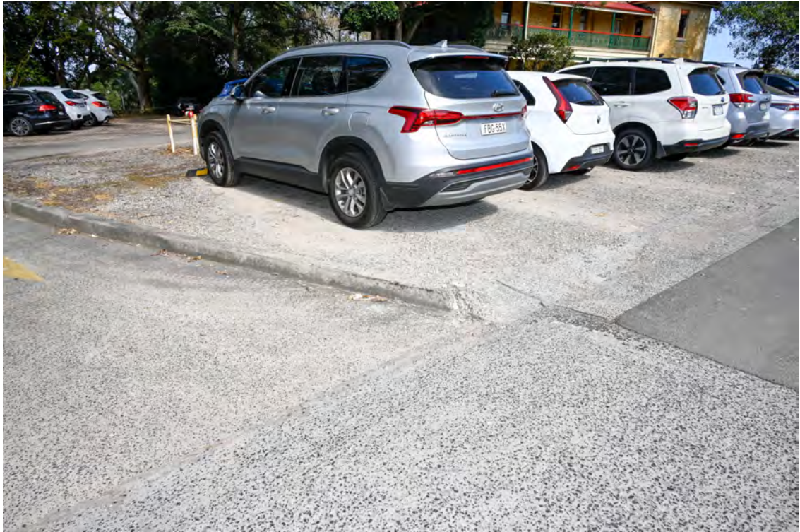
Hospital access road from St Vincents Road. Area of Pallister House. Damaged kerb.
