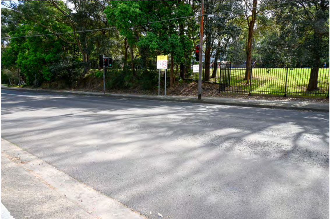
Internal access road on the western side of the hospital building. Intersection with River Road. Cracked and crazed road paving.
