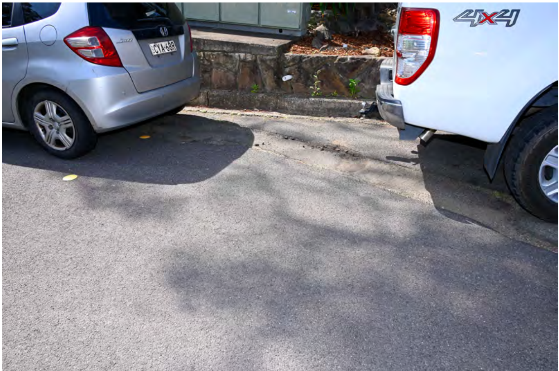
River Road. Area of the proposed substation works. Area on the eastern side of the internal access road. Damaged road paving.
