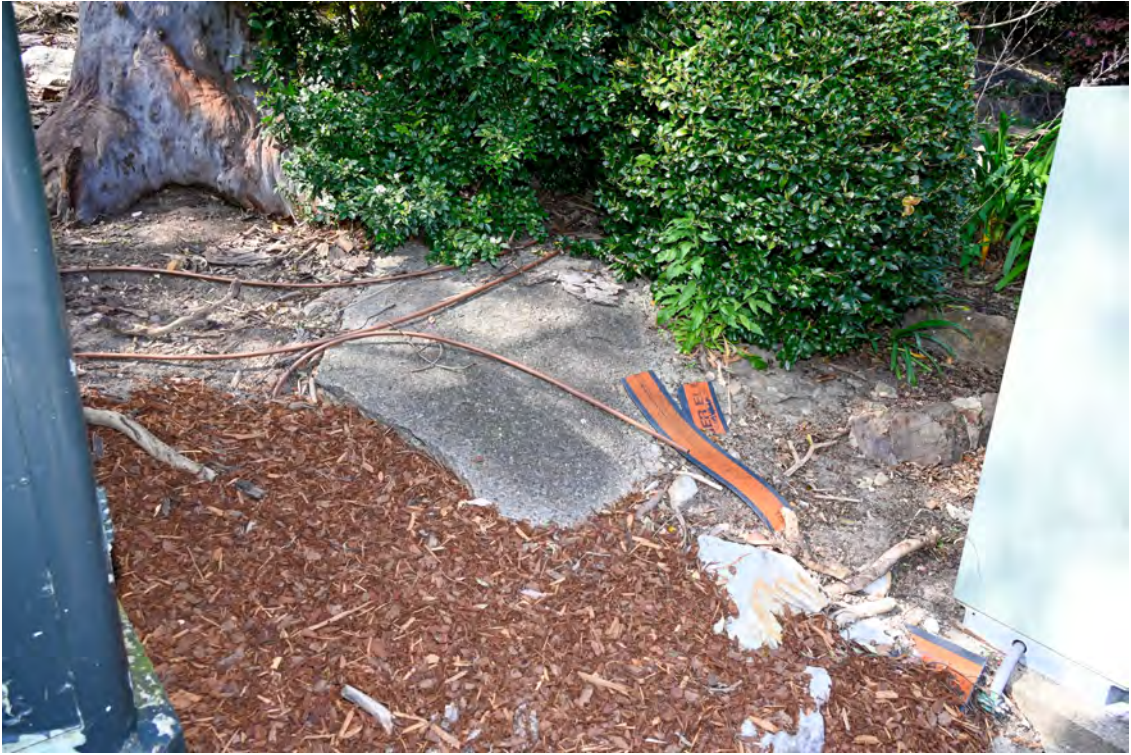
River Road. Area of the proposed substation works. Area on the eastern side of the internal access road. Record of the landscaping.
