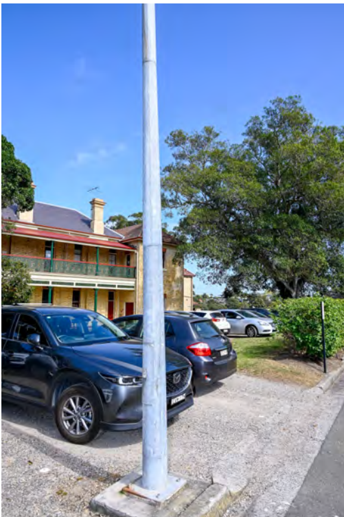
Internal road adjacent to Pallister House. Heading west. Light pole.
