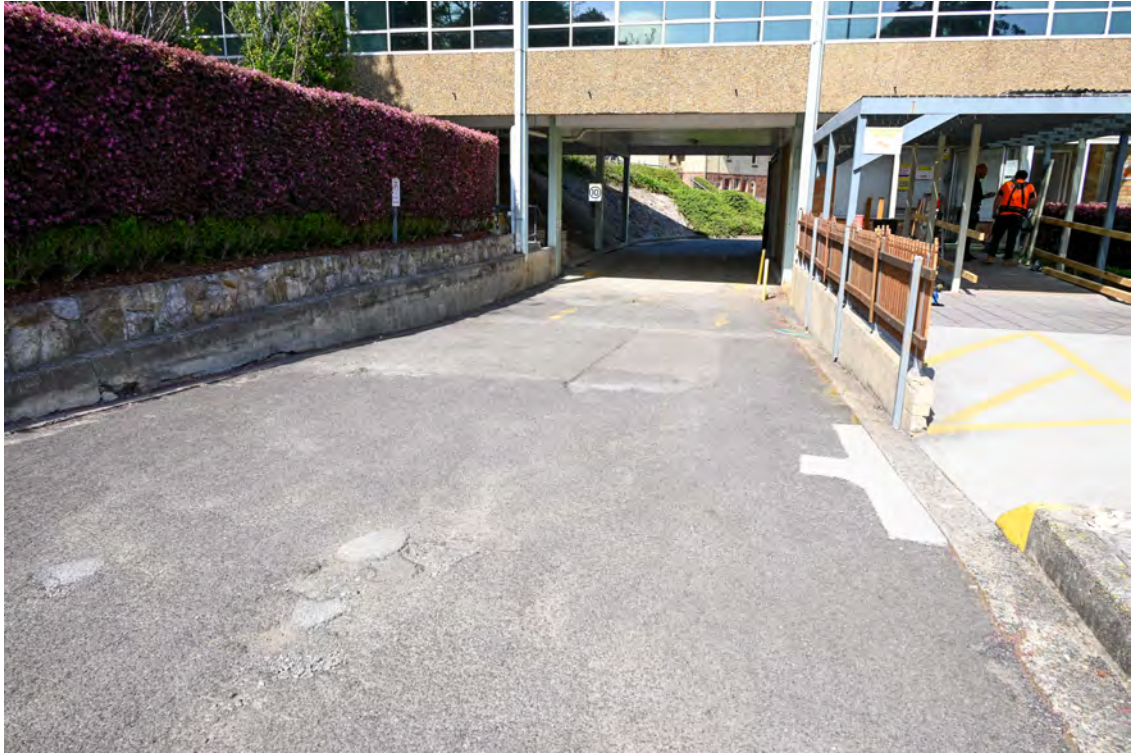
Internal access road from River Road. Heading south approaching the overhead walkway. Damaged road paving.
