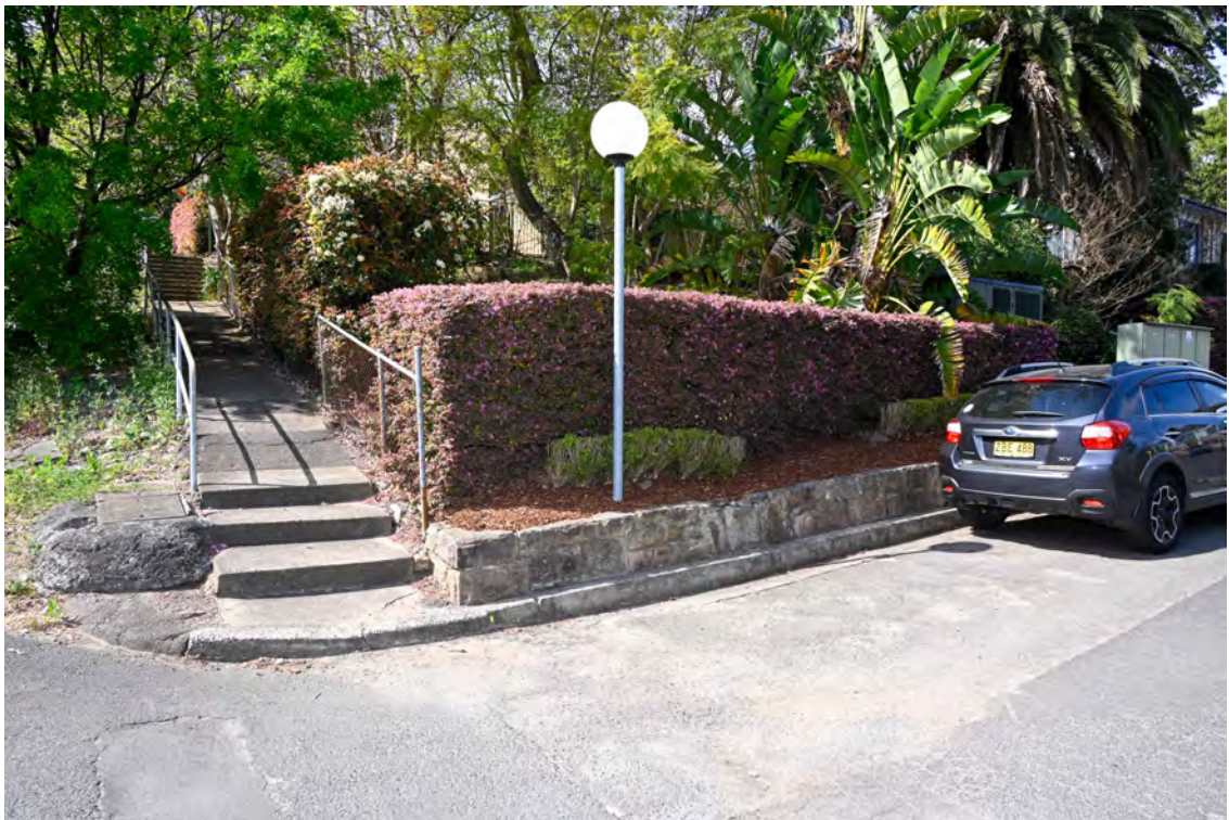
River Road. Area of the proposed substation works. Area on the eastern side of the internal access road.
