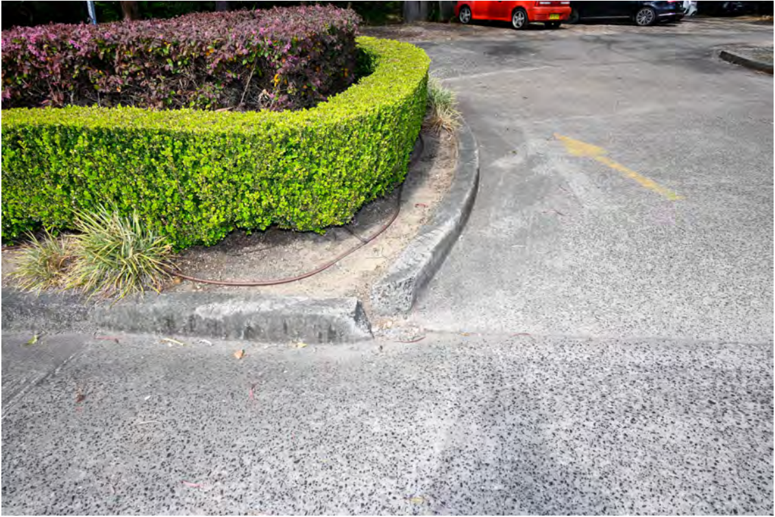
Hospital access road from St Vincents Road. Access / exit to Pallister House. Damaged kerb.
