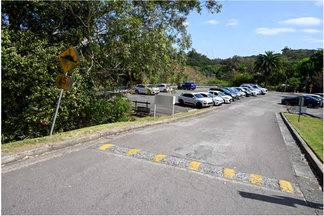
Western side of the property. Internal access road. Heading north towards River Road. Damaged road paving.
