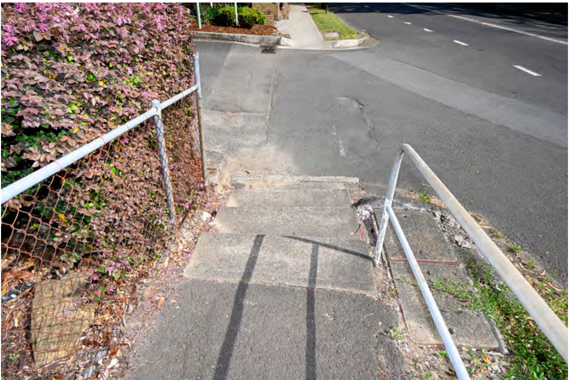
Hospital access from River Road. Area of the proposed substation works. Heading west. Footpath / steps.
