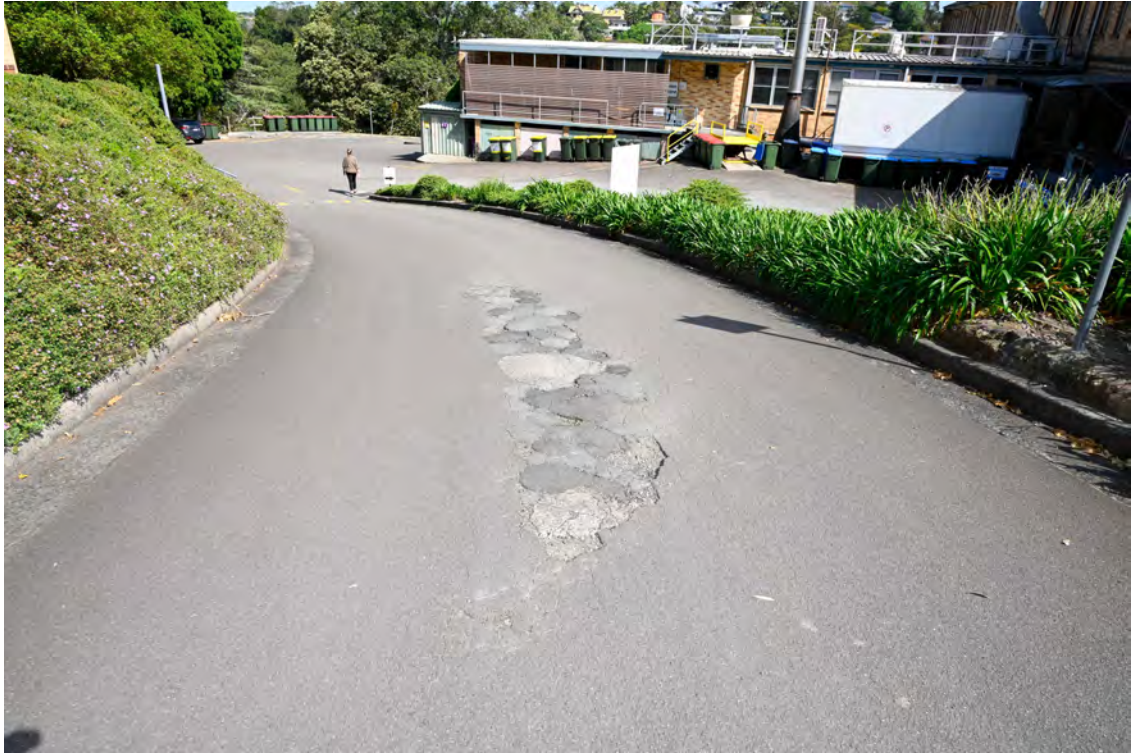
Internal road between Pallister House and 'Health & Care'. Heading south-west / downhill. Damaged road paving. Area of proposed road works.
