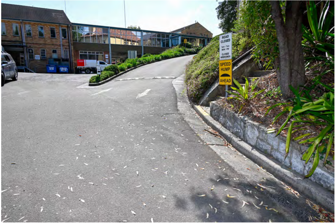
North-western side of Pallister House. Area of proposed road works. Facing north-east / uphill.
