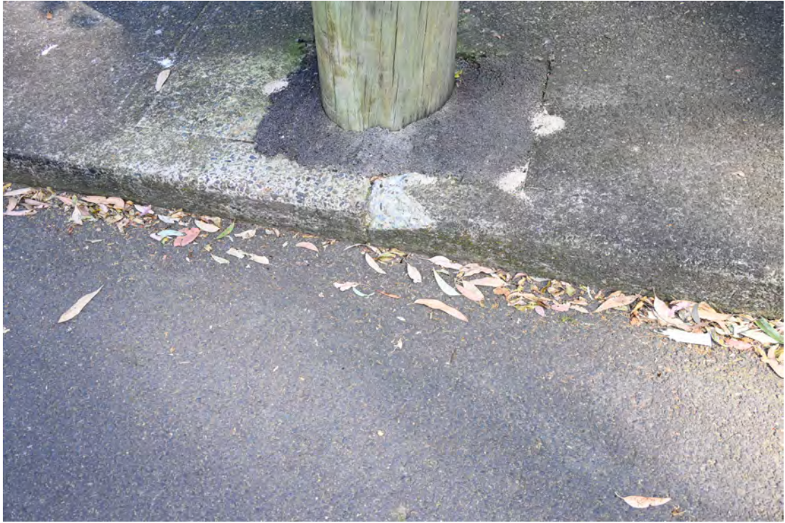
Hospital access from St Vincents Road. Northern side of the intersection with the access road. Power pole no. GL72349. Chipped kerb.
