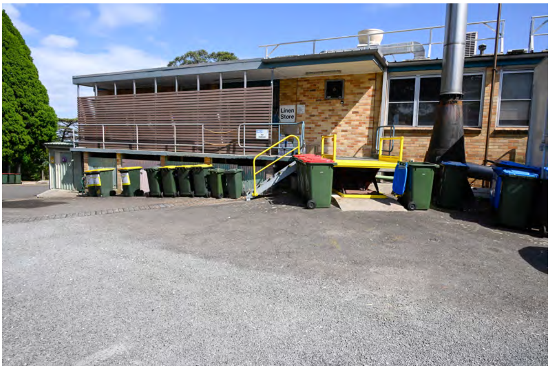
Internal access road. Heading south. Area of 'Service and deliveries'. General record of the area.
