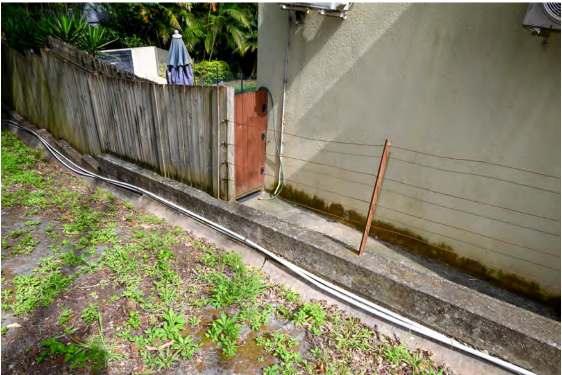
Western hospital boundary. Heading south. Area adjacent to the common boundary with 117 River Road.
