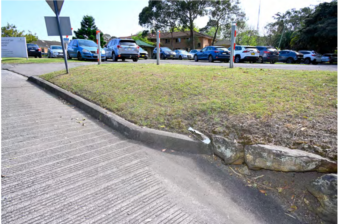
Hospital access road from St Vincents Road. Heading west / uphill towards Pallister House. Damaged PVC drain pipe.
