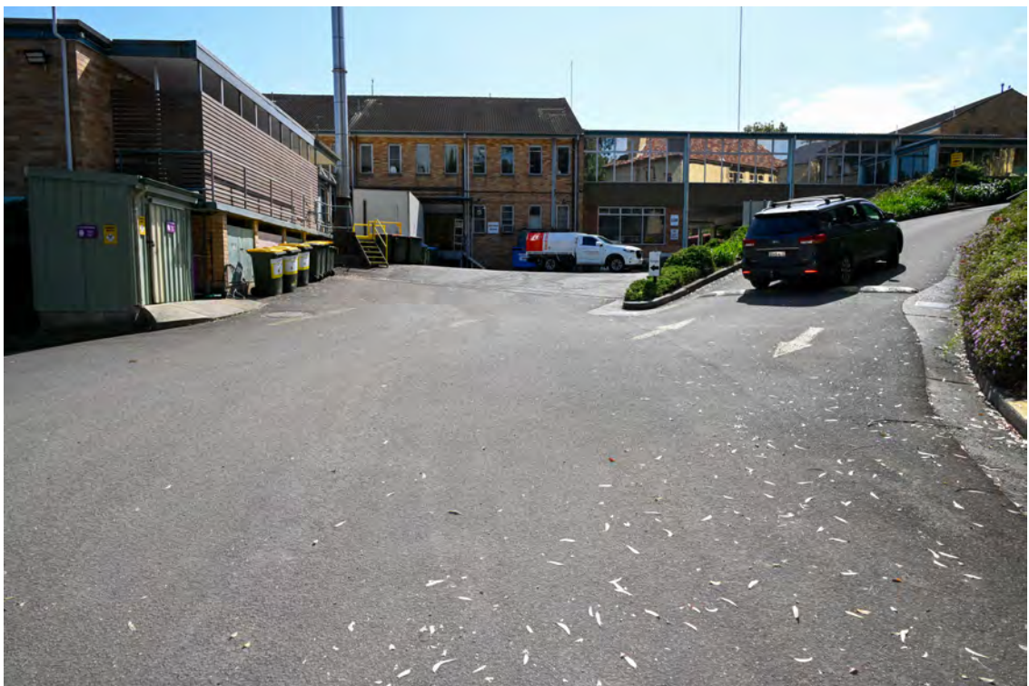
North-western side of Pallister House. Area of proposed road works. Facing north-east / uphill.
