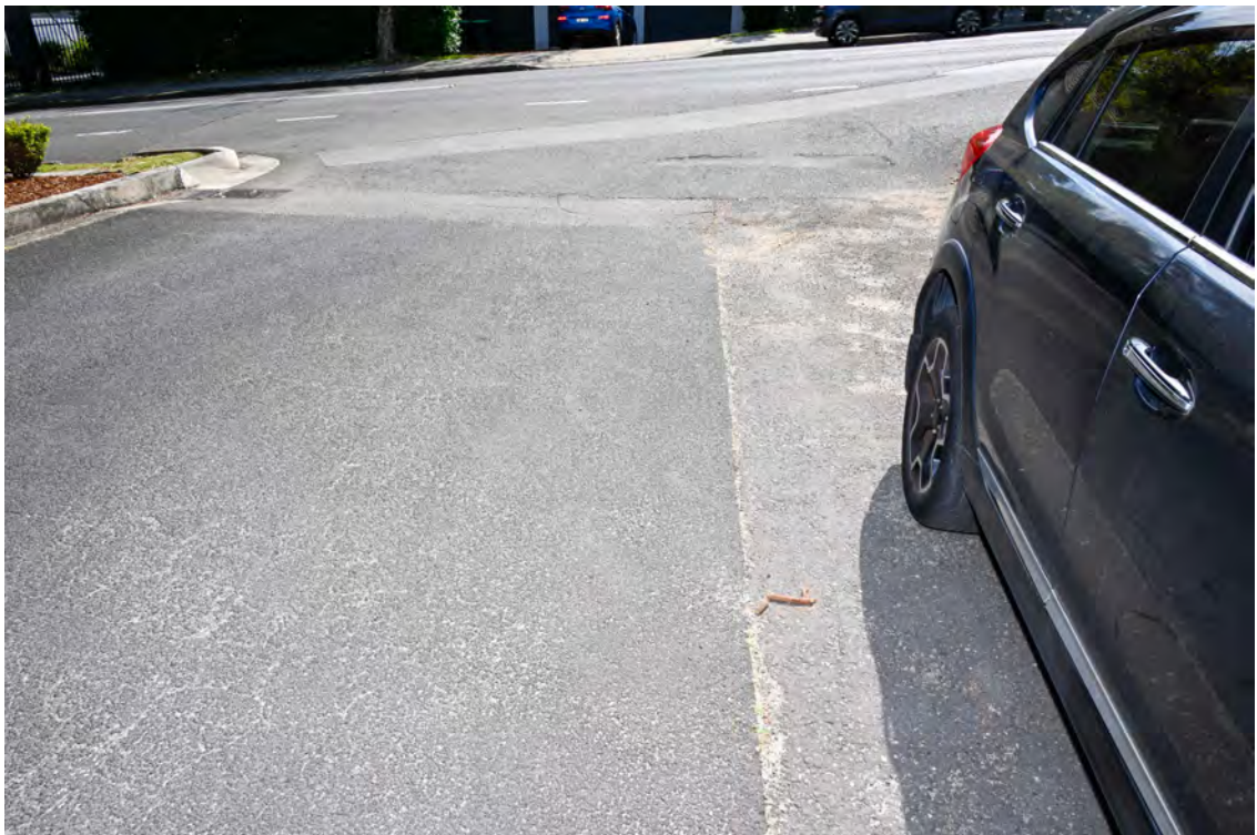
River Road. Area of the proposed substation works. Adjacent internal access road. Heading north towards River Road. Cracked and crazed road paving.
