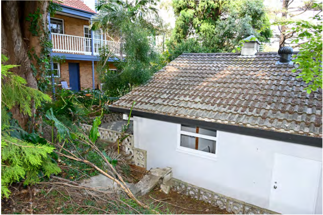
Southern property boundary. Heading east towards St Vincents Road. Common boundary with 24 Gore Street.
