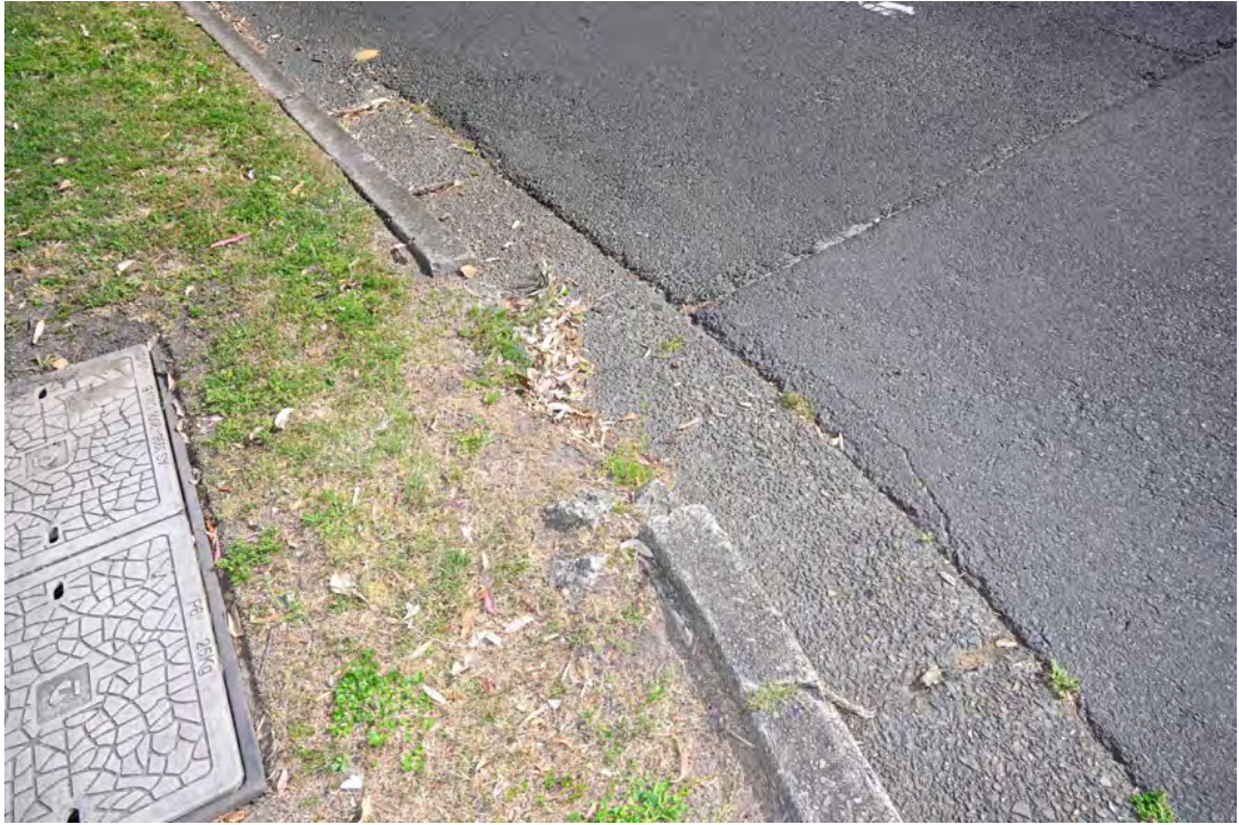
Hospital access from River Road. Area of the proposed substation works. Western side of the intersection. Heading west. Area of the 'Sprinkler Booster'. Damaged curb.
