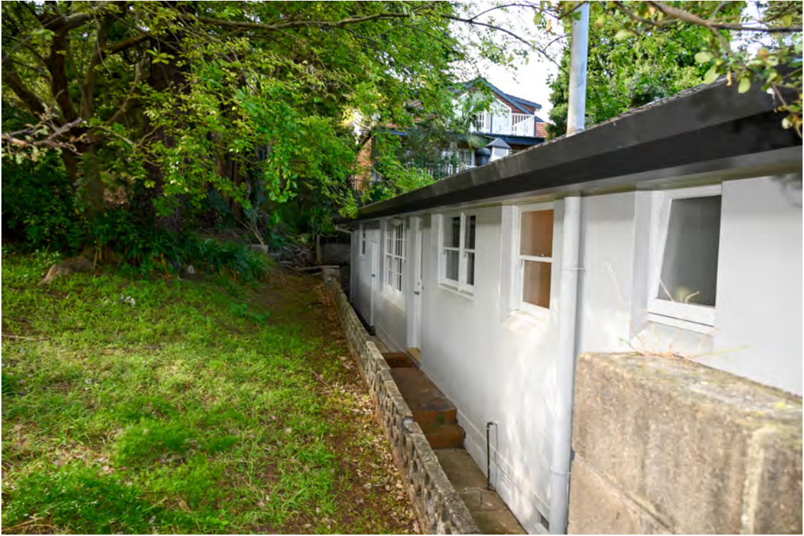
Southern property boundary. Heading east towards St Vincents Road. Common boundary with 24 Gore Street.
