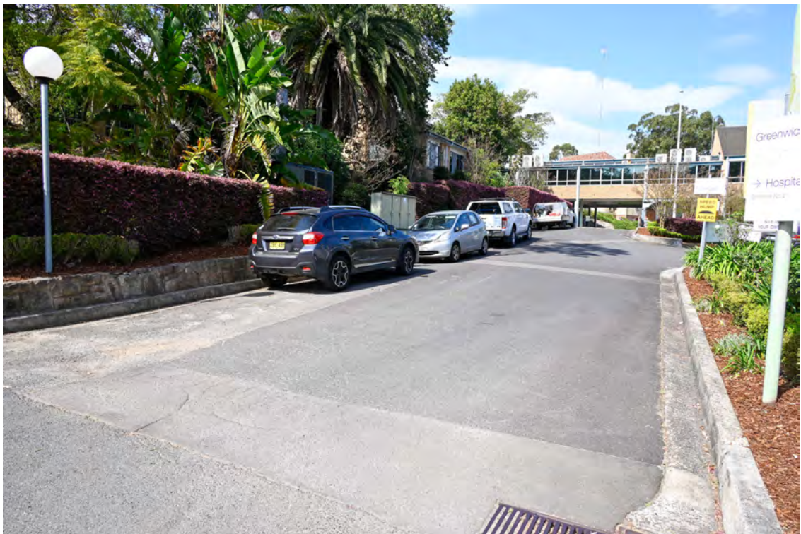
Greenwich Hospital access from River Road. Area of the proposed substation works.
