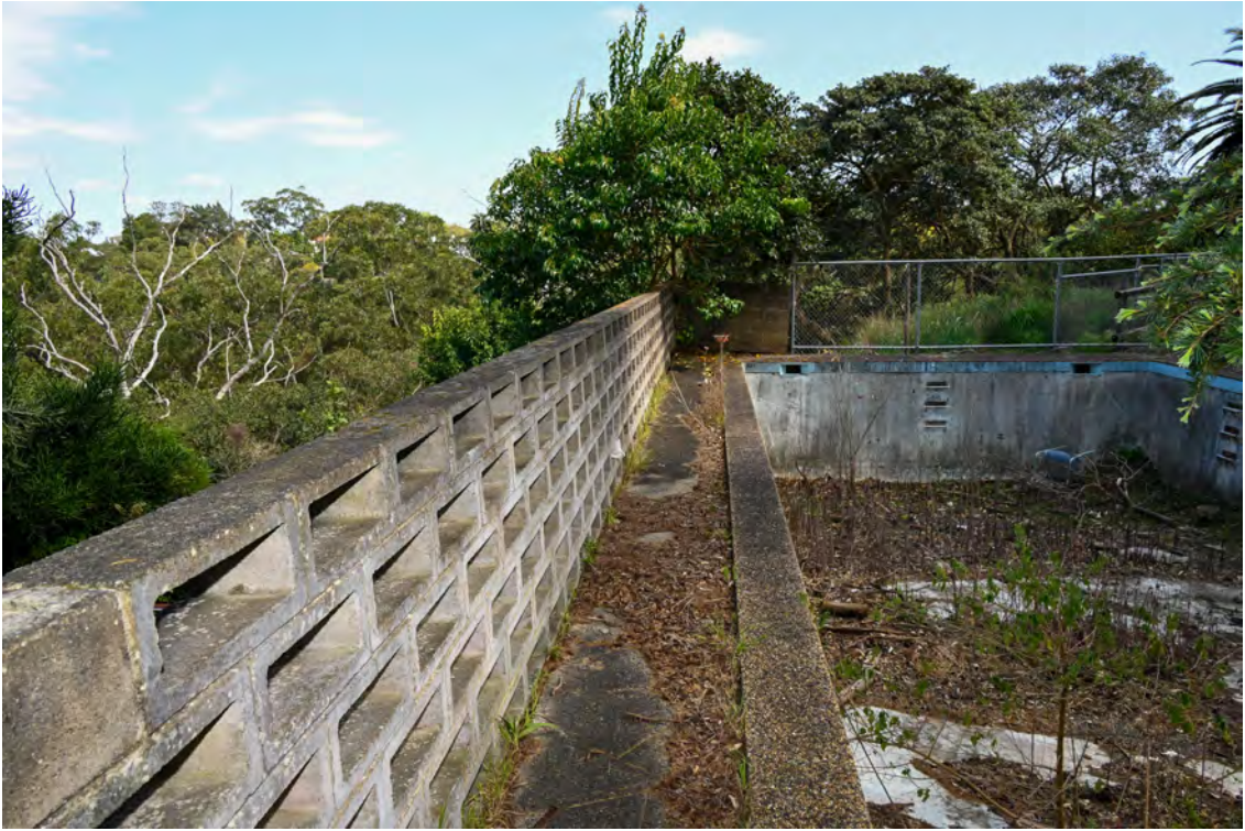
Southern property boundary. Heading east towards St Vincents Road. Breeze block breeze block boundary wall to the unused swimming pool.
