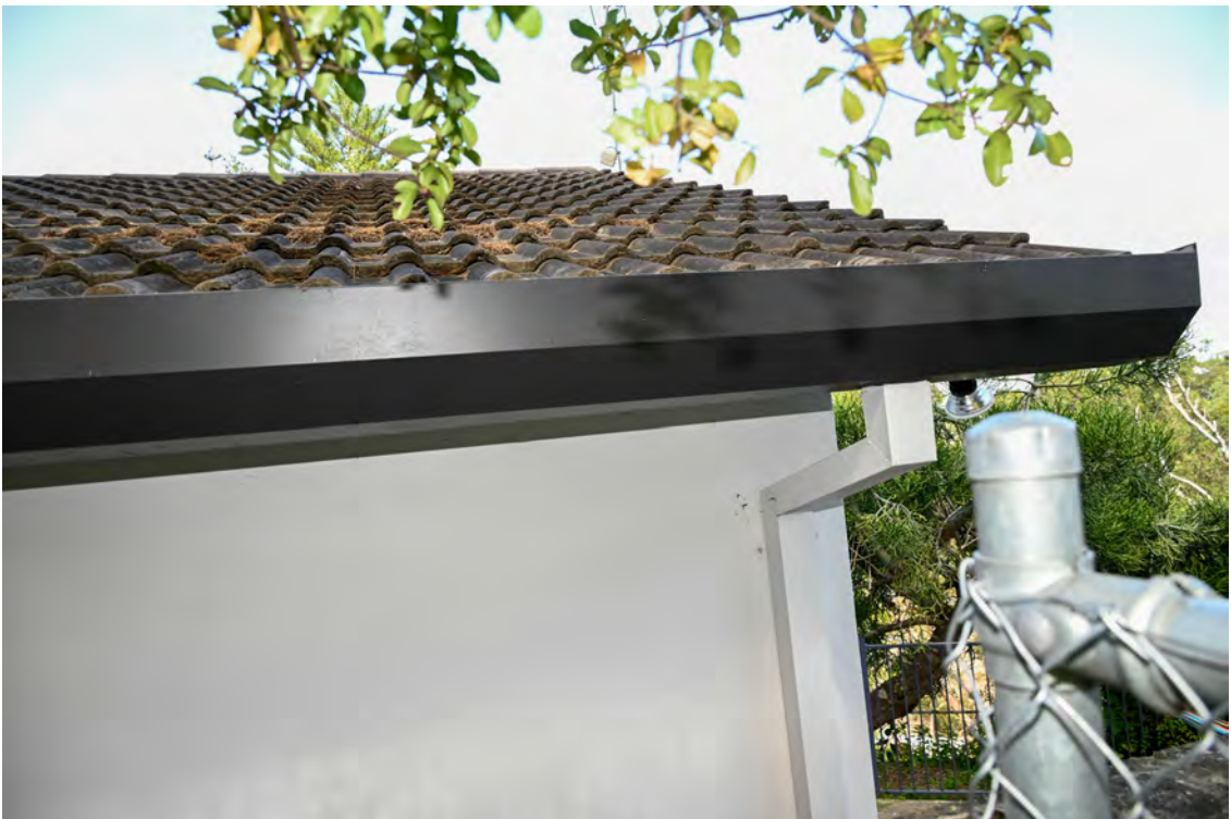
Southern property boundary. Heading east towards St Vincents Road. Common boundary with 24 Gore Street.
