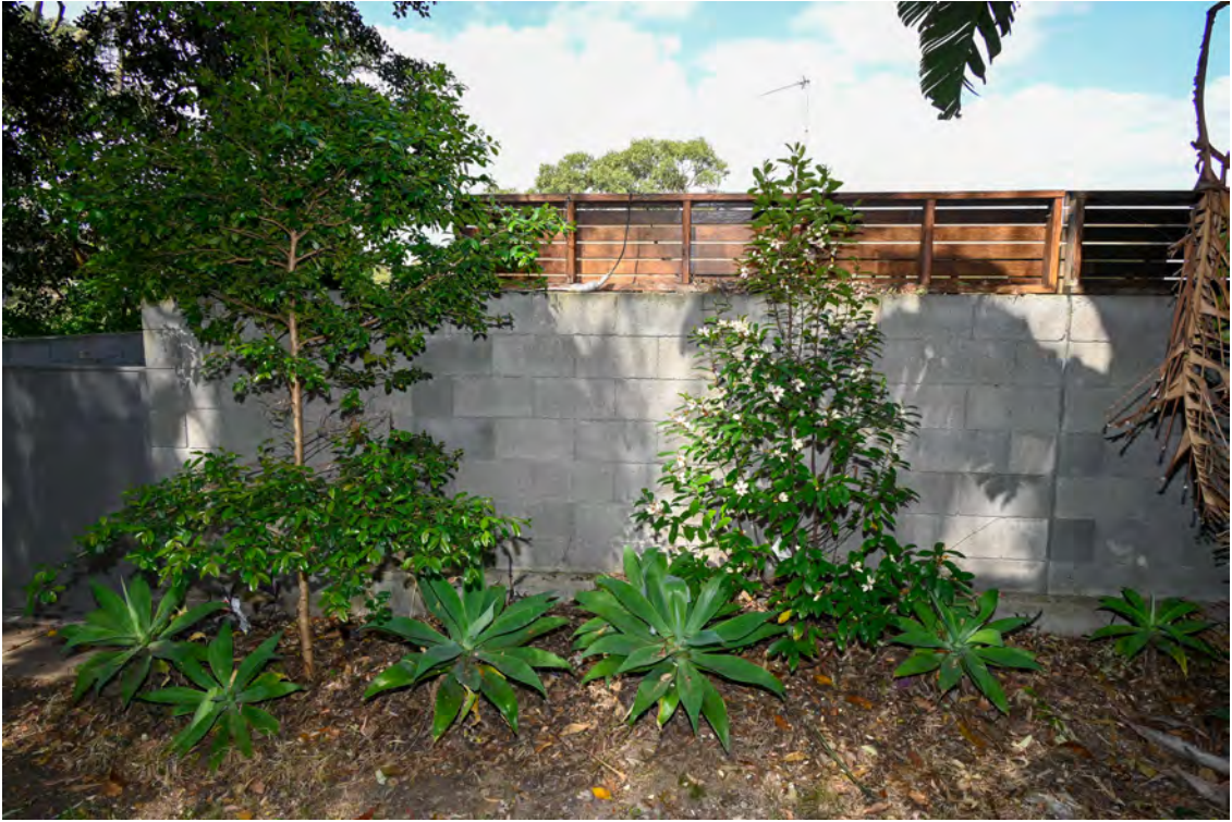
Southern property boundary. Heading east towards St Vincents Road. Common boundary with 51-47 Gore Street.
