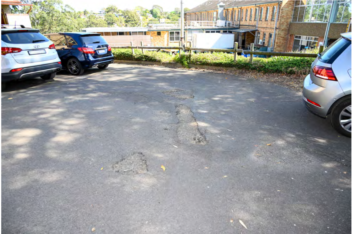
Area on the northern side of Pallister House. Adjacent car parking area. Damaged paving.
