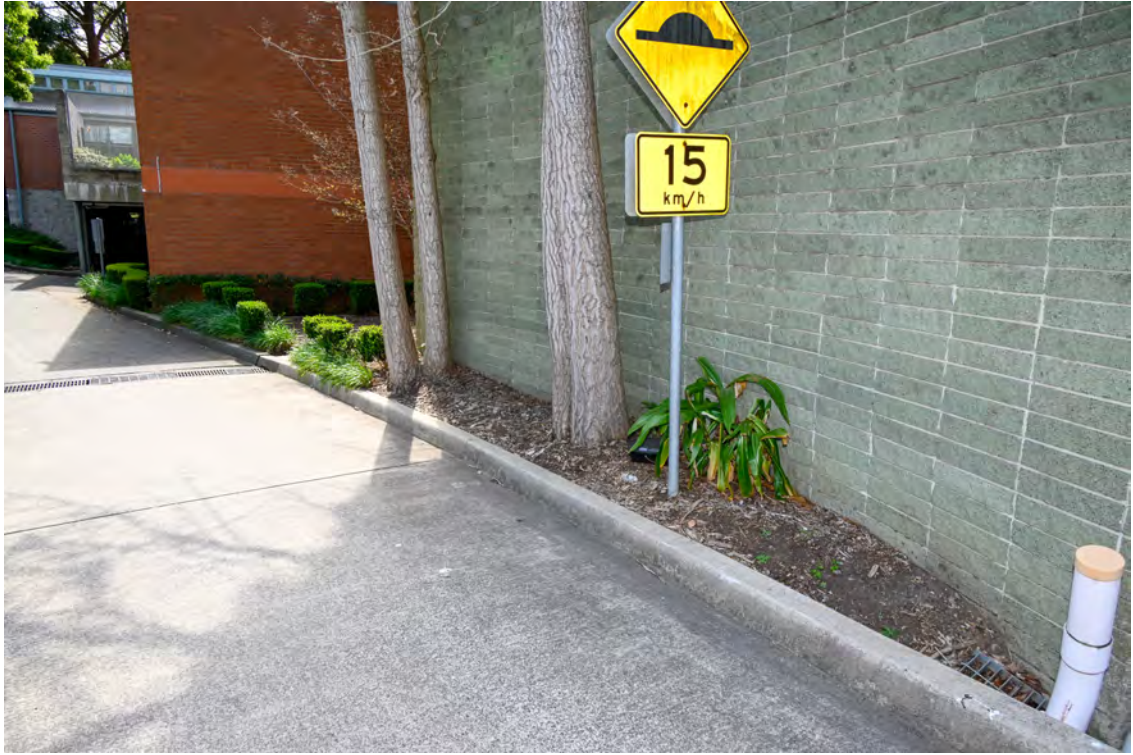
Western side of the property. Internal access road on the western side of the hospital building. Heading north towards River Road.
