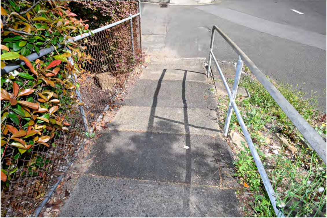
Hospital access from River Road. Area of the proposed substation works. Heading west. Footpath.
