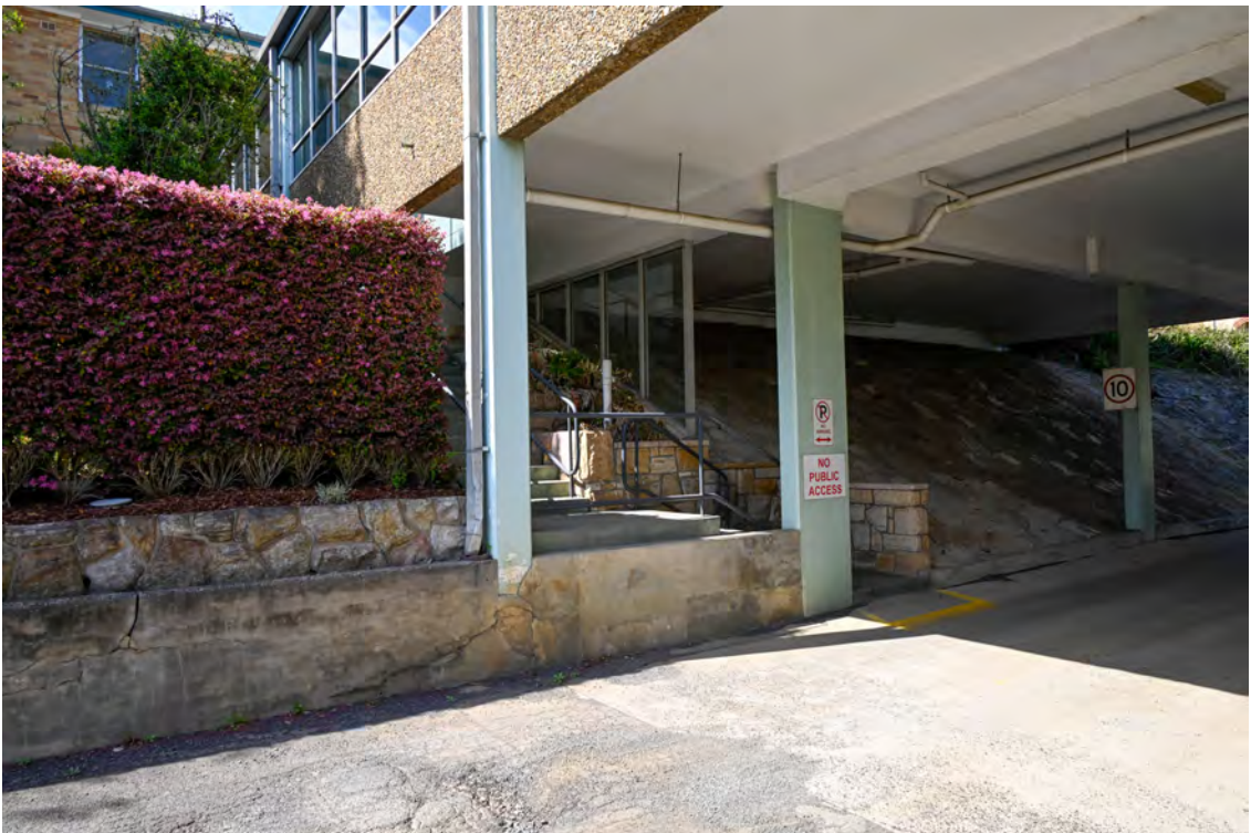
Internal access road from River Road. Heading south through the 'tunnel'. Eastern side.
