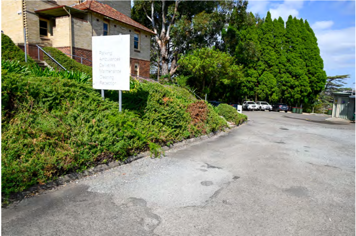
Internal access road. Heading south. Area of 'Service and deliveries'. Retaining structure below the area of road works. Damaged road paving.
