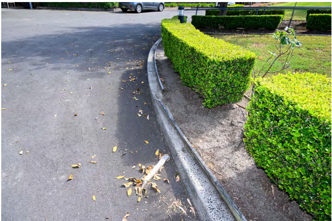
Internal road adjacent to Pallister House. Heading west. Damaged timber edging.
