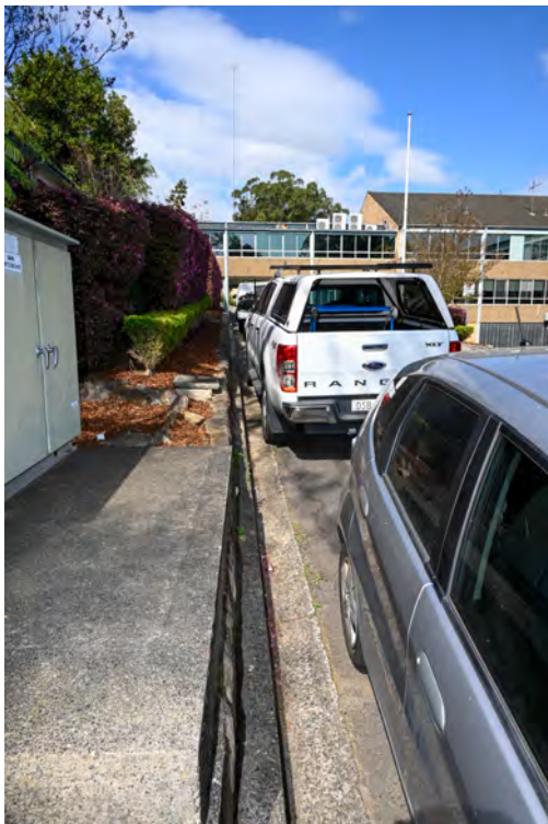
River Road. Area of the proposed substation works. Area on the eastern side of the internal access road. Stone retaining wall.
