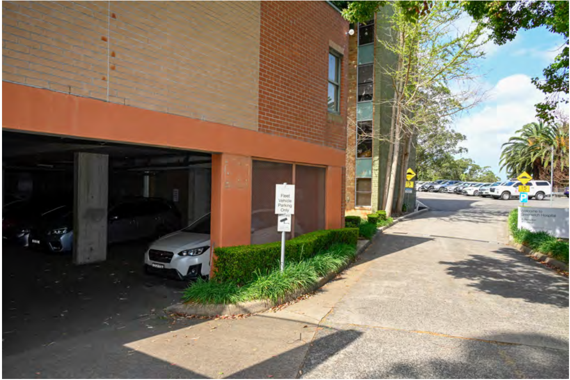
Western side of the property. Internal access road on the western side of the hospital building. Heading north towards River Road. Structure above the undercover parking.
