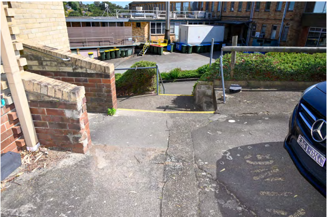
Area on the northern side of Pallister House. Adjacent car parking area. Steps leading down to the area of road works.
