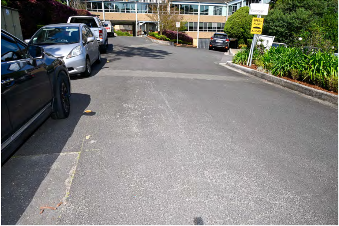
River Road. Area of the proposed substation works. Internal access road. Cracked and crazed state of the road paving.
