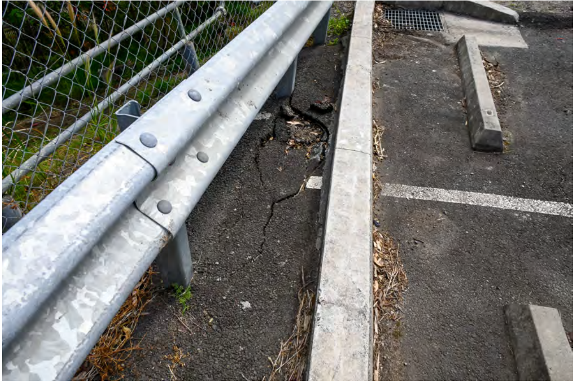
Western hospital boundary. Heading south. Area adjacent to the common boundary with 117B River Road. Subsistence to the paving.
