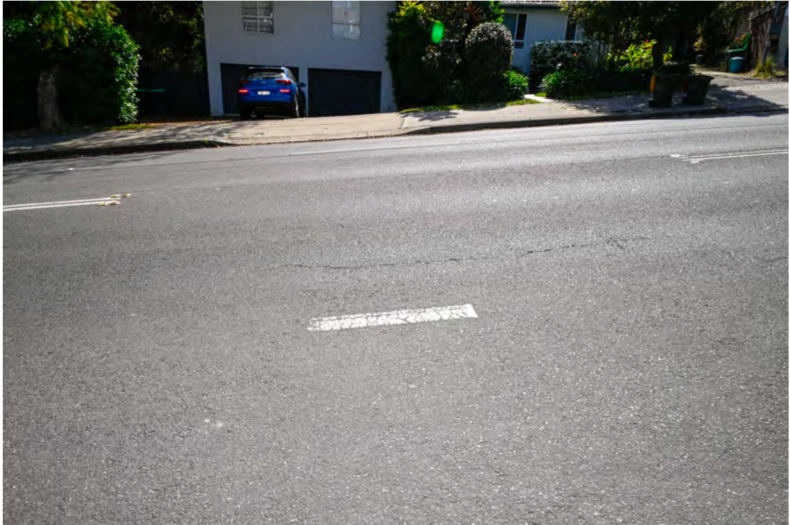
Hospital access from River Road. Area of the proposed substation works. Heading east. Cracked road paving.
