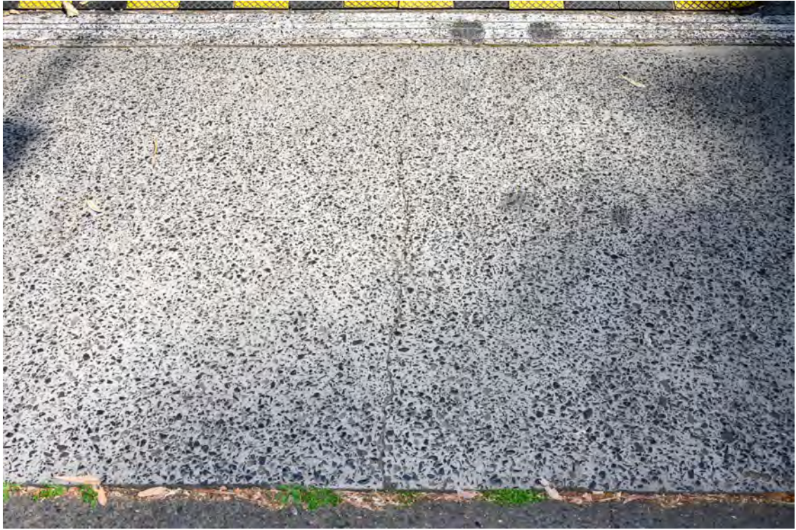
Hospital access from St Vincents Road. Intersection with the access road. Cracked paving.
