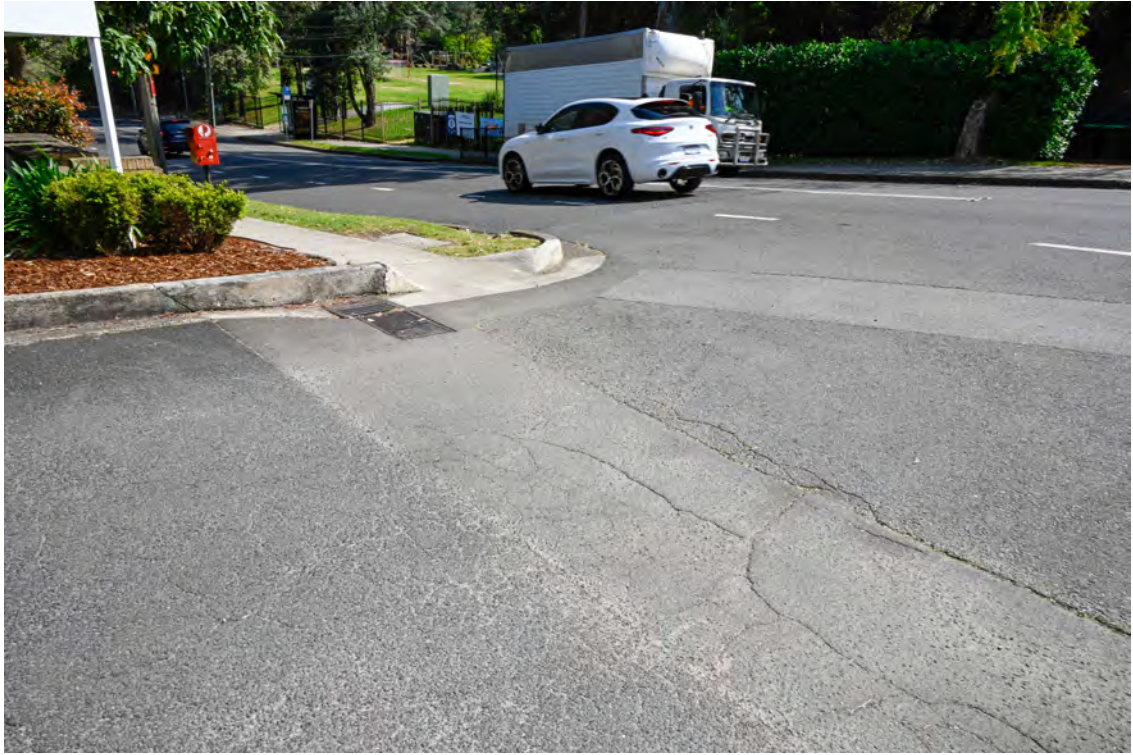
River Road. Area of the proposed substation works. Adjacent internal access road. Heading north towards River Road. Cracked paving.
