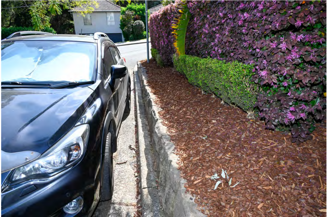
River Road. Area of the proposed substation works. Area on the eastern side of the internal access road. Stone retaining wall.
