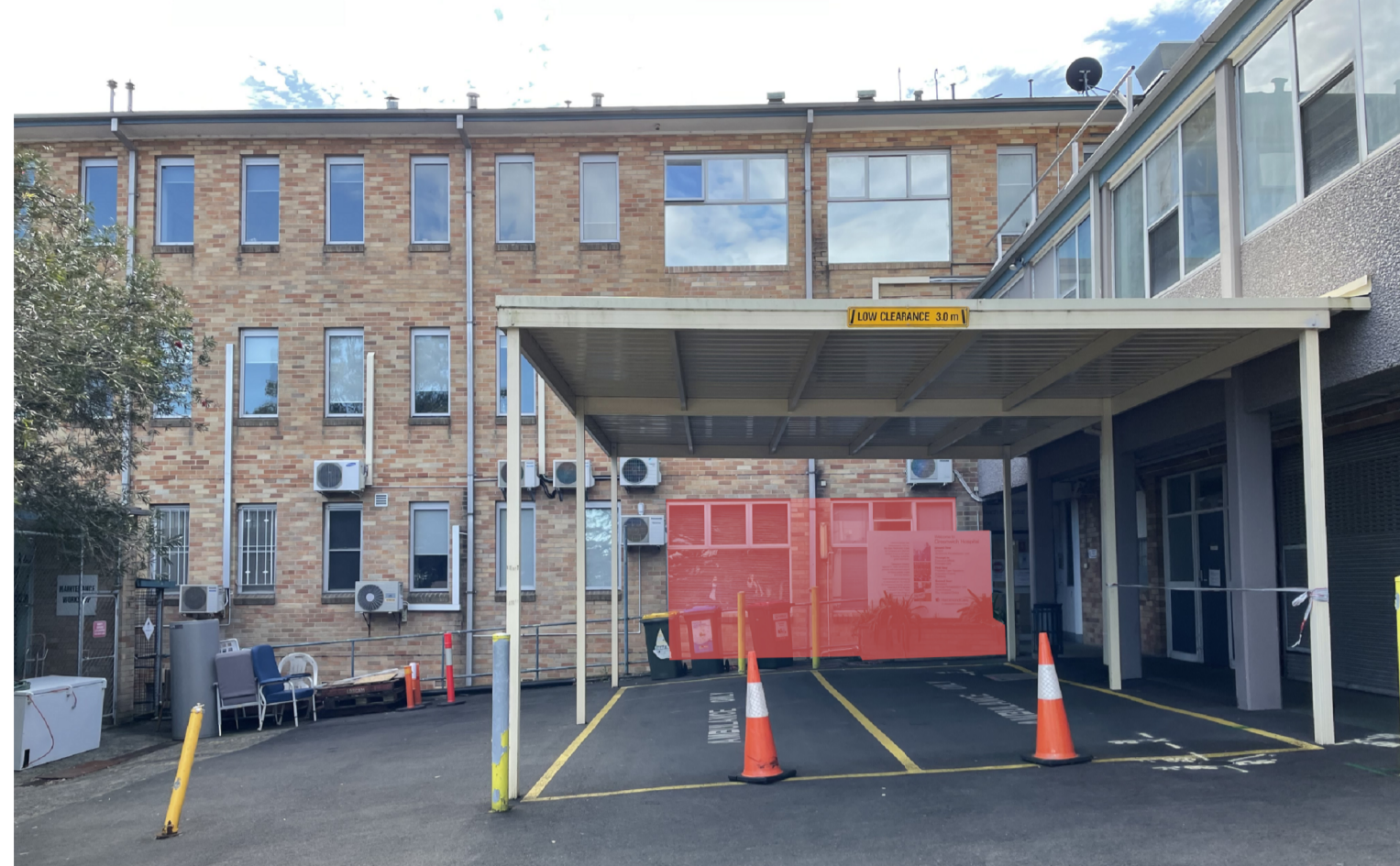
VIEW P1: RED HIGHLIGHTED AREA OUTLINES PART OF BUILDING TO BE DEMOLISHED IN STAGE 1
