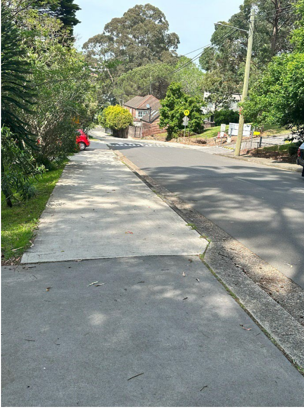
Photo 2 – Existing 2.0m All Weather Path Eastern Side St Vincents Road with Marked Footcrossing South of Driveway Access
