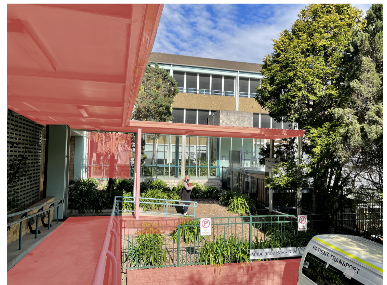
VIEW P3: RED HIGHLIGHTED AREA OUTLINES PART OF BUILDING TO BE DEMOLISHED IN STAGE 1
